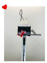
Have you ever been stranded at home because you had lost power and your car was stuck in the garage because the garage door wouldn't open? It's worth knowing how to bypass the automatic part and do things manually if the need arises... \*\*\*Do not disconnect power while the door is up. If you happen to have a broken spring, the full weight of the door could come crashing down, smashing anything in its path, as well as ruining your garage door (and those aren't cheap!!)\*\*\*
